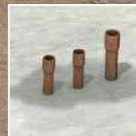
Leaking Penetrations i.e. Pipe Penetrations
