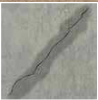
Leaking Cracks
